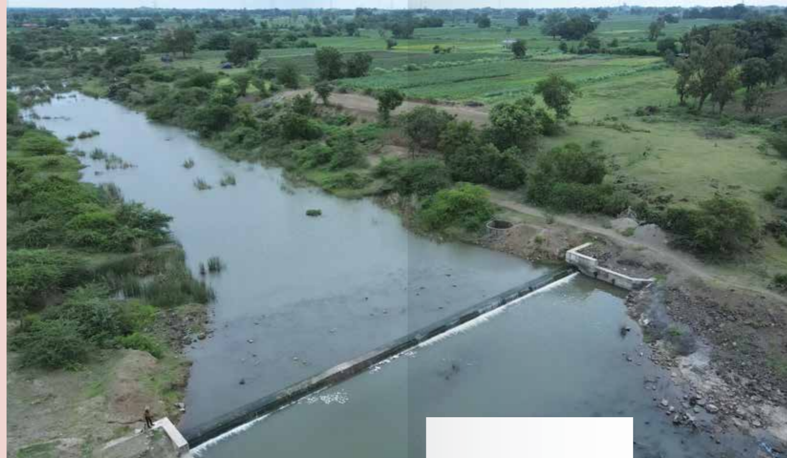
Zanjhmer check dam developed in collaboration with Narmada, Water Resources, Water Supply and Kalpsar Department of the Government of Gujarat
